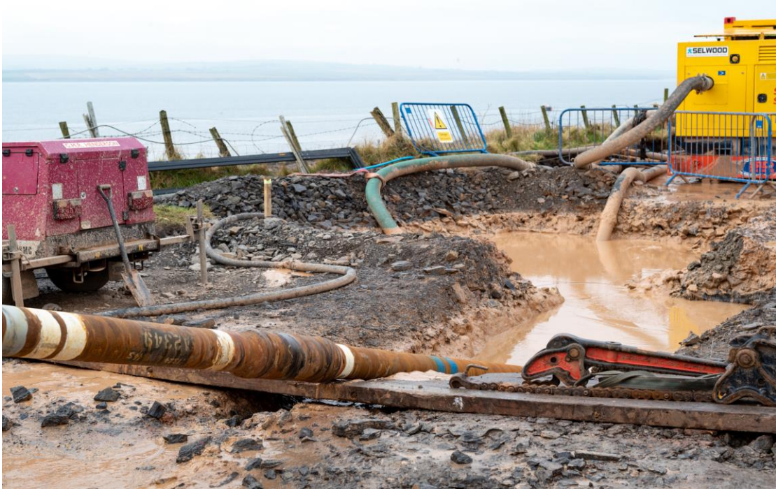
Figure 6 Example of HDD entry pit
